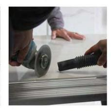
Cutting the panels can require special equipment. If a hole is required, then a standard diamond core bit can be used. If a full-length straight cut is required, then a special cutting table and snap cutter is suggested. Using the correct equipment will ensure clean, straight edges and a quality installation.
